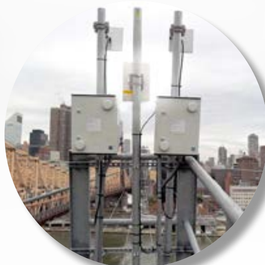
2. DATAEAGLE Classic 3702A in the protection cabinet at one of the two cabins.
